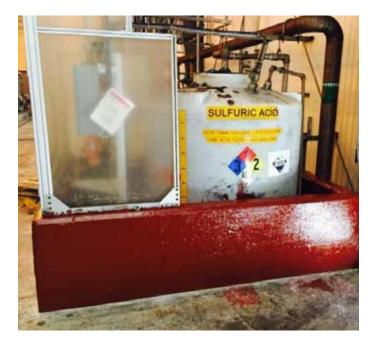
Belzona 4361 is a flexible barrier coating for the protection of chemical containment areas.
