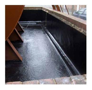
Belzona 4351 is a two-component, static dissipative coating designed to transfer surface build-up of electrostatic charge away from hazardous areas. Due to its excellent static dissipative properties, Belzona 4351 helps to eliminate the chances of electrostatic charge as an ignition source where flammable materials are stored.
